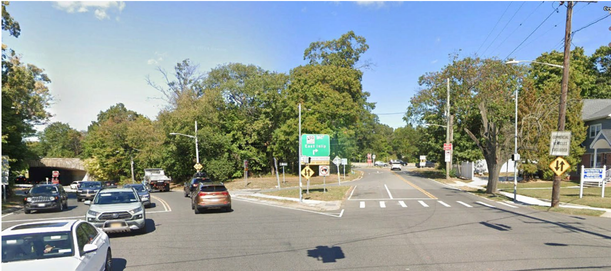
View from Central Avenue facing the underpass and east-bound ramp to SSP.
