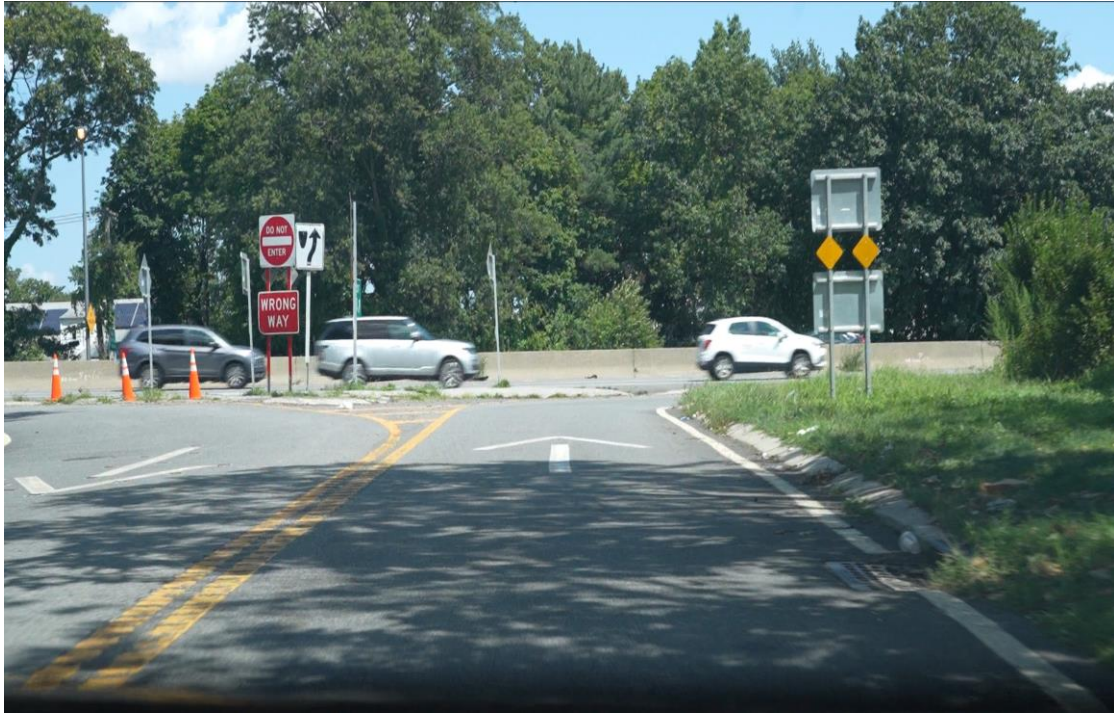
Figure 13: Central Avenue Leading to Southern State Parkway.
