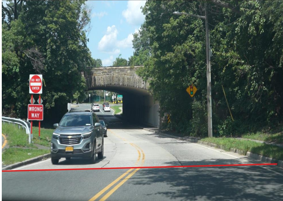
Figure 10: Central Avenue Approaching Linden Boulevard
