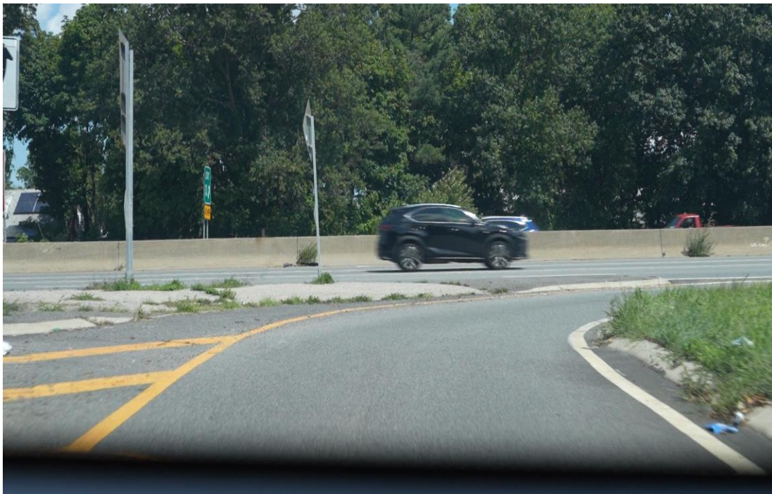
Figure 14: Central Avenue Leading to Southern State Parkway.
