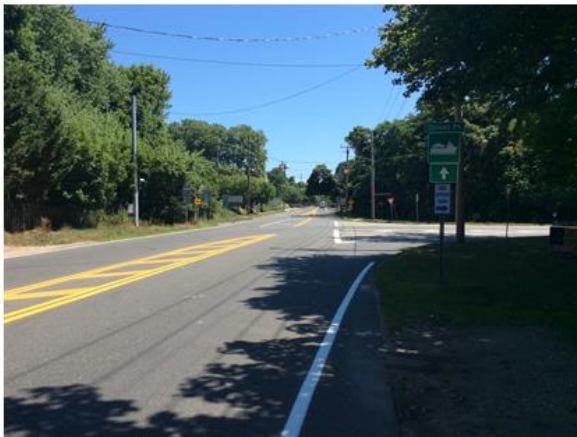
Eastbound Approach (CR48 / North Road)
