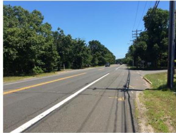
Southbound Approach (NY 114)
