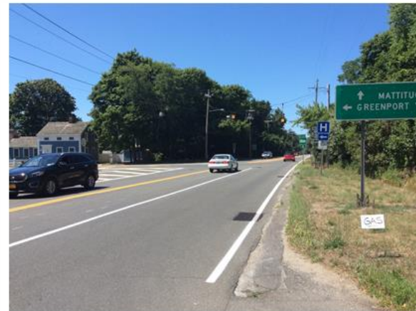
Westbound Approach (NY 25/Main Road)
