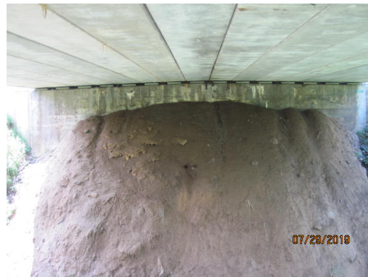
Begin Abutment under Bridge (Looking South)
