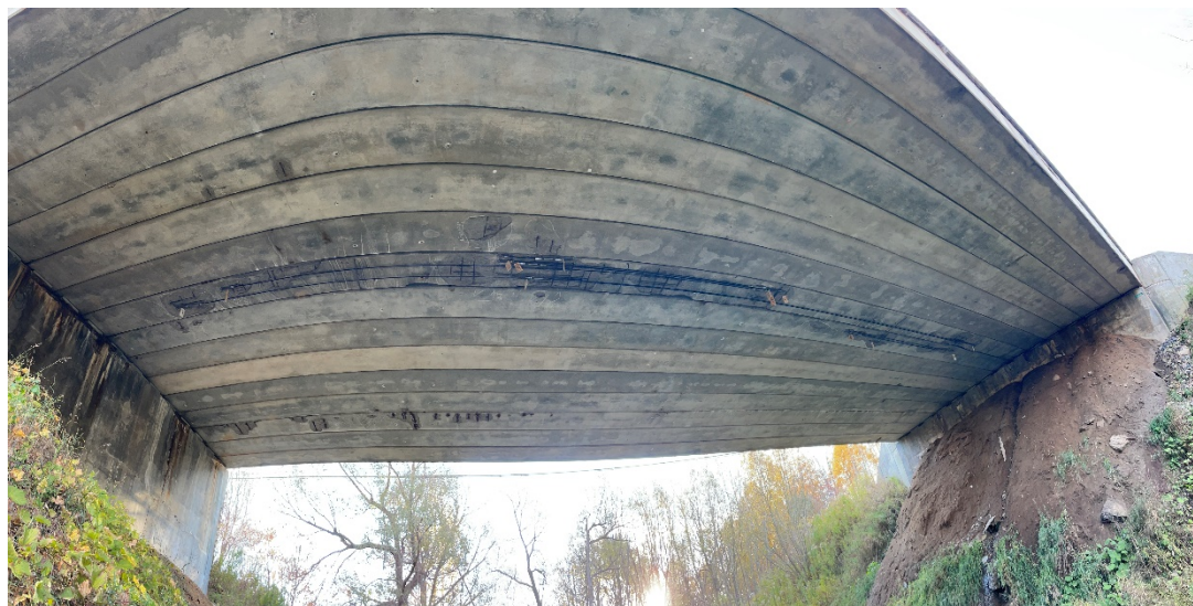
Bridge Superstructure (Looking East)
