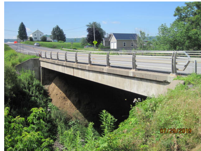
East Bridge Elevation (Looking Southwest)
